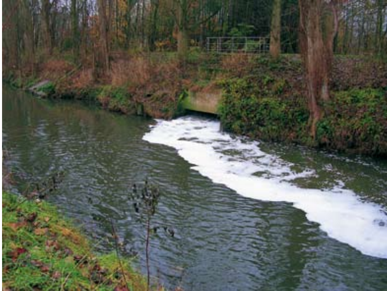
A very vivid substance flow: outlet of the wastewater treatment plant in Beggen
