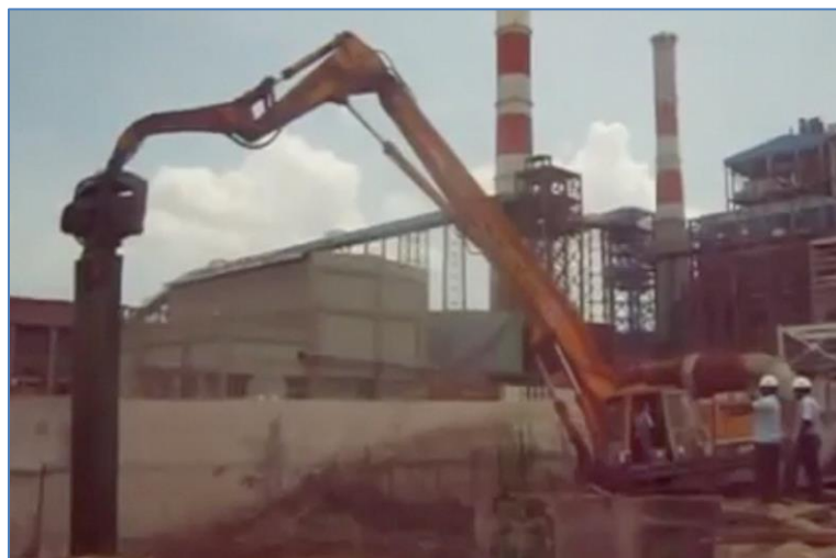
Figure 10.10: Sheet pile removal for reverse logistics and re-renting. Source unnamed YouTube.
