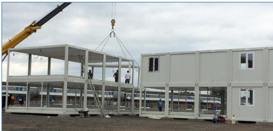
Figure 10.11: Circularity in practice. Modular steel units being constructed from recycled steel. Source Modular Construction Solutions GmbH.
